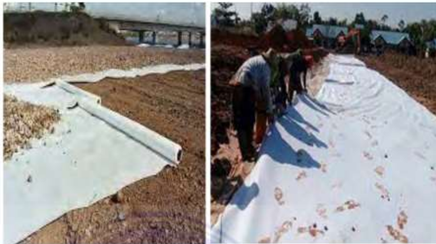
Gambar 2. Proses penghamparan geotextile
