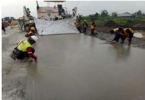
Gambar 4. Proses curing beton
